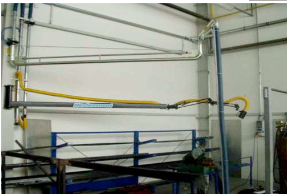
Working place of weldment grinding.
