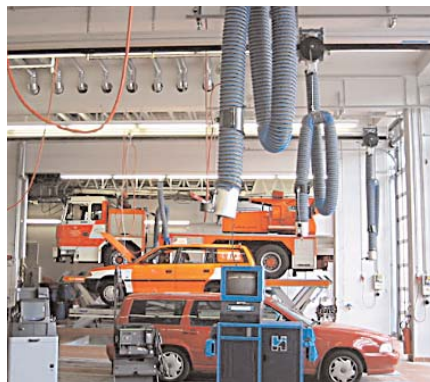
The Vehicle maintenance shop with Exhaust Rail System ALU 150
